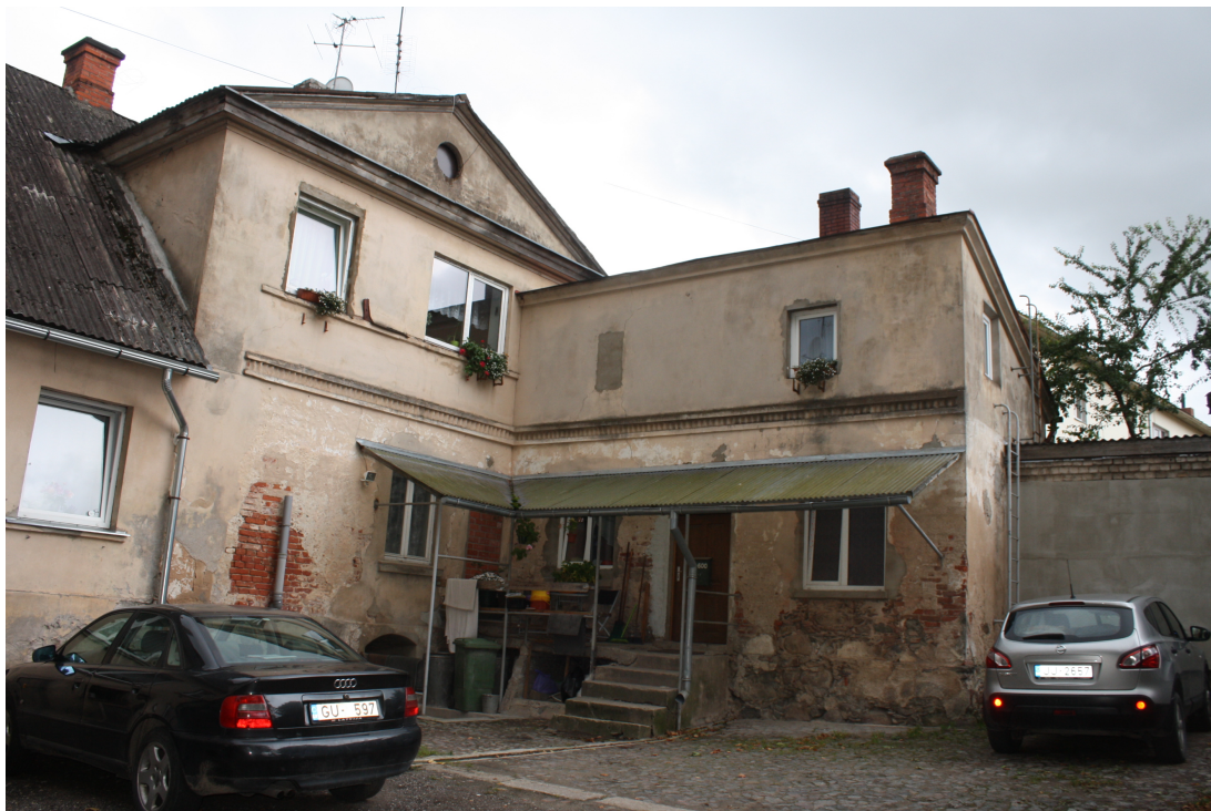
Laidzes_4_88010120080001_fasade7 Pagalma fasādes fragments.
