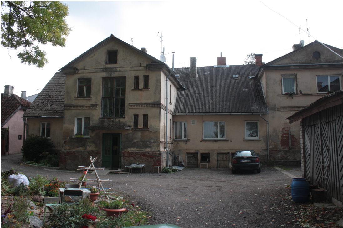
Laidzes_4_88010120080001_fasade5 Pagalma fasādes fragments.
